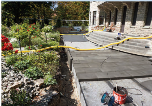
Employees of the company GFI Baumanagement, Oetzberg near Frankfurt/Main, specializing in concrete repair and masonry drying during the insulation of the exterior walls of the library of Haus Cramer.
