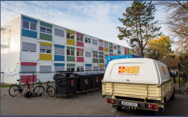
“Container village” in Berlin-Zehlendorf, managed by the Arbeiter-Samariter-Bund (ASB). In 2016, the Berlin Senate plans to build 24.000 modular dwellings for refugees at 60 different locations and infrastructure which can be used both by local residents and refugees.
