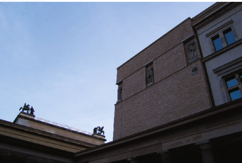
Back view of the Neues Museum with roof of the Altes Museum .
