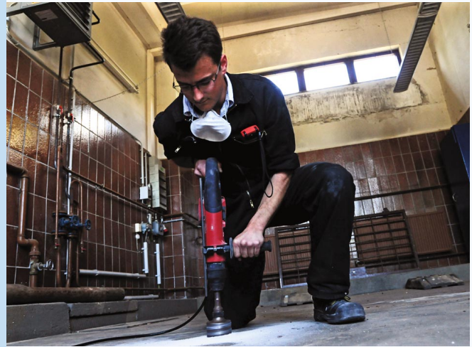
Chris Stiedemann (Civil and Environmental Engineering), Berlin student in spring 2008, at the Gesellschaft für ökologische Bautechnik , Berlin, conducting a test drilling.
